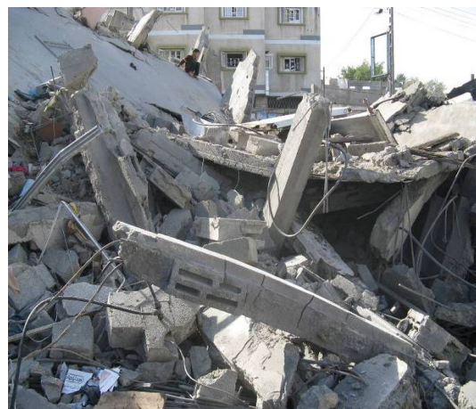
Demolished Shijai'a Clinic- January 2009
